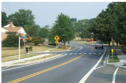
Lane Striping to Narrow Travel Lanes
